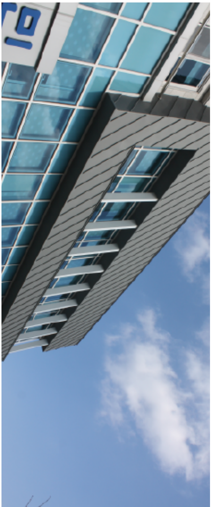
Vertical and horizontal standingseam joint
