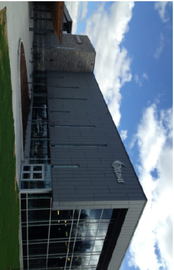
Vertical and horizontal roll formed panel joint
