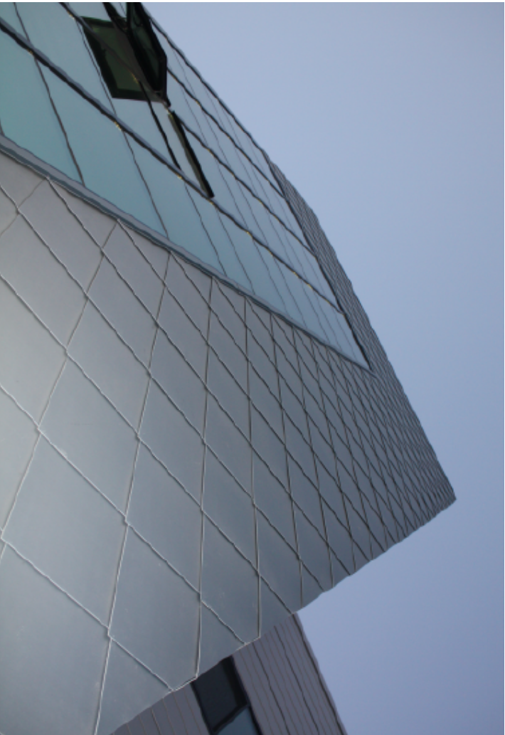
Vertical and horizontal flat lock joint
